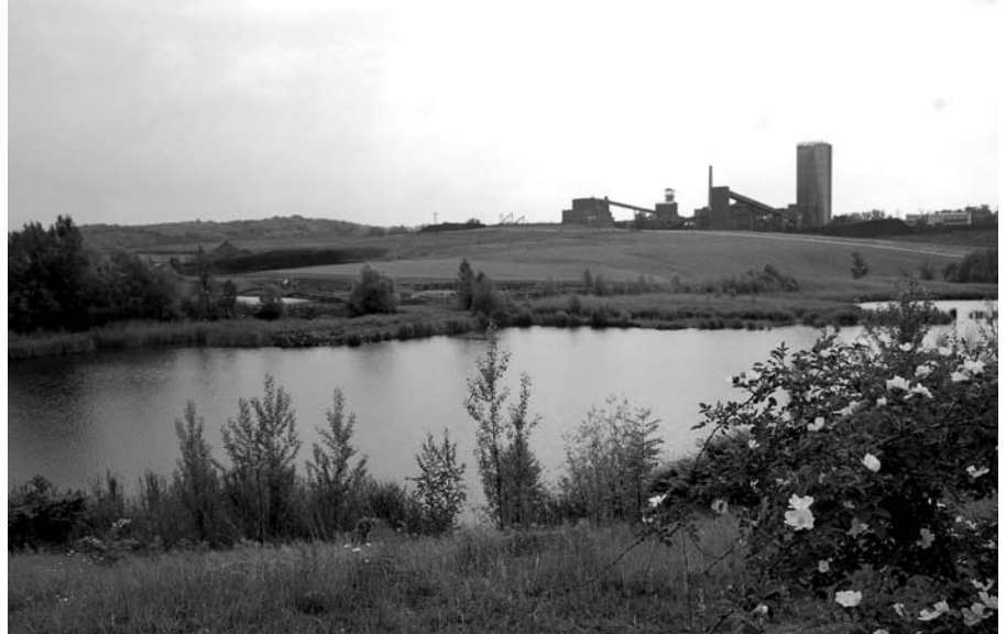
Rehabilitation project – Lazy settling reservoirs in Karviná
